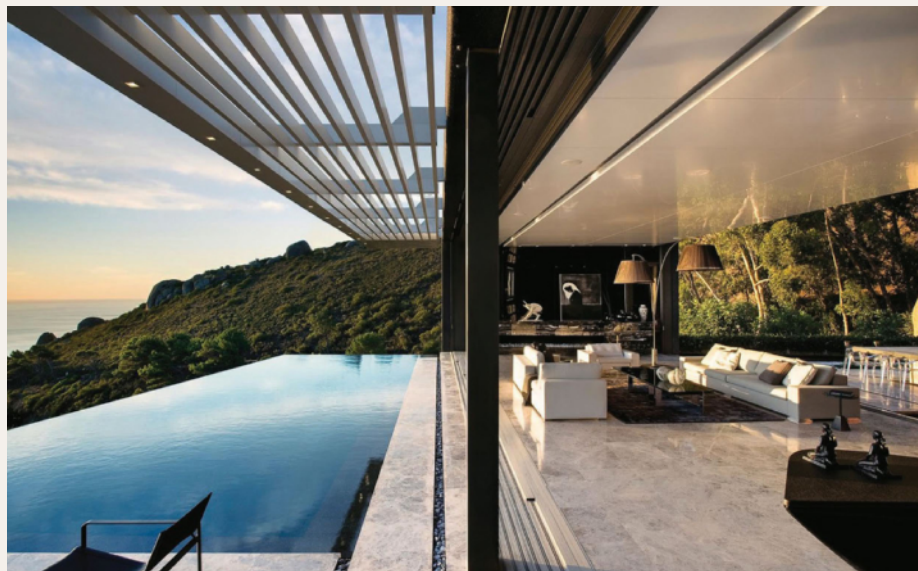
Clifton Beyond is designed to take full advantage of the views out to the ocean
